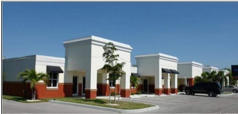
The office building in Ft. Myers
